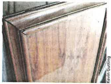
Among the Victory's features getting needed TLC: the mahogany woodwork shown partially restored here.
